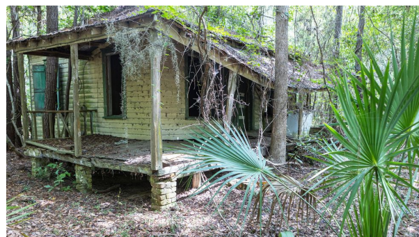
Traditional Gullah house on stilts.
